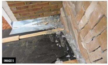
The metal flashing is reverse-shingled over the brick, which can lead to leaks.
