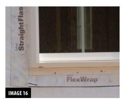
The sill flashing was correctly installed before the window.
