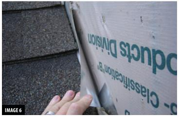
The housewrap was improperly installed behind the step flashing, allowing water that gets behind the siding to run down the housewrap and penetrate between the step flashing and housewrap. This will lead to a ceiling leak.
