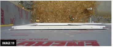
Water running down a wall "sees" an entry point as it approaches the head of a window. The window head must be properly sealed and flashed to avoid water entry.
