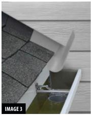
Premolded, seamless, kick-out diverter flashing is available in multiple colors. This product is manufactured by DryFlekt.
