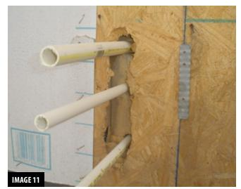
The lack of flashing around the pipes coming through this wall will allow water to run down the pipes and flow directly into the wall.
