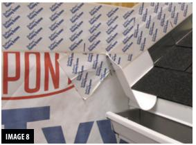
This is a properly integrated, seamless, kickout diverter flashing with peel-and-stick flashing and housewrap.
