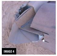
Metal kick-out diverter flashings often are poorly field-fabricated, which can lead to leaks.
