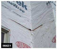
The rips and gaps in this housewrap will allow water flowing behind the cladding to leak into the wall at the corners.
