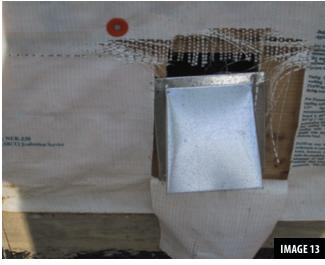
Cutting holes that are larger than necessary to accommodate penetrations, like this vent, defeats the purpose of a housewrap.
