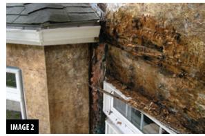
Water damage easily can occur at roof-wall intersections when flashing is neglected.
