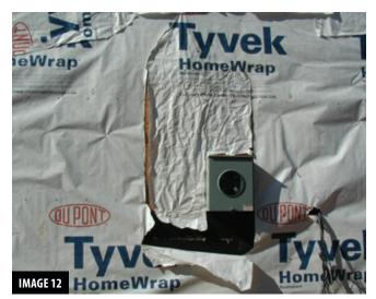
Poor detailing at the electric-meter base will eventually lead to leaks.
