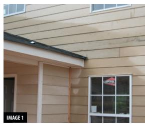
There is obvious moisture buildup at this roof-wall intersection. The contractor should have installed kick-out diverter flashing.
