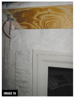
Proper sequencing will ensure a window is watertight. In this final step of installation, the head flashing should be installed from the nail fin at the window head onto the wall sheathing.
