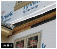
The large gaps in the WRB at the roof-wall intersection certainly will lead to a failure. Housewraps should cover walls completely and be properly lapped to shed water.
