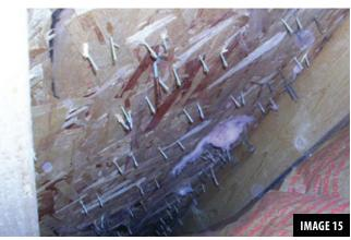
A housewrap can be over-fastened. Every staple through a WRB is a potential water leak. Wrap caps are a better option.
