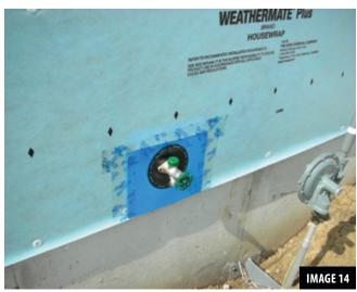
A prefabricated flashing device stretches around pipes and seals them. This product is manufactured by QuickFlash.
