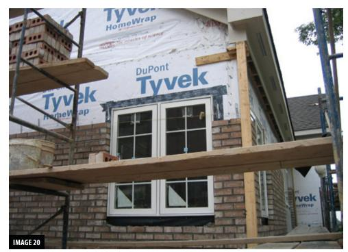
The head flashing on the window is reverse lapped over the housewrap.
