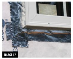
The sill flashing is improperly applied over the top of the nail fin below the window. In a correct installation, the sill flashing should be installed before the window.
