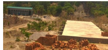
EWB science lab foundation, note handmade bricks Boys ablution block, background
