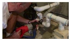
Figure 6. A reciprocating saw often works well to cut PVC pipe during the installation process.
