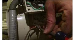
Figure 8. Make sure the ground bonding wire is securely fastened to the pump's bonding lug.
