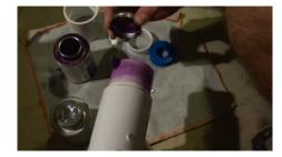
Figure 7. Thread sealant or pipe glue will help ensure fittings remain connected and leak-free.
