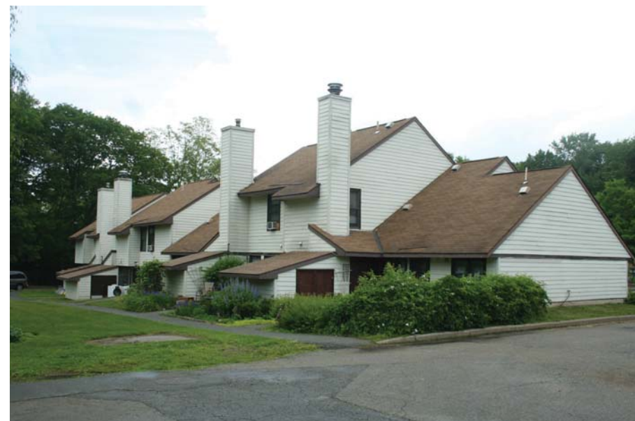
8. Each apartment has an outdoor storage and mechanical room extending off the back, with semi-private terrace space in between for each unit. Many are pushed up fairly close to the rising landscape. They appear to be well-used amenities. The chimneys are used to vent the heating and hot water systems.
