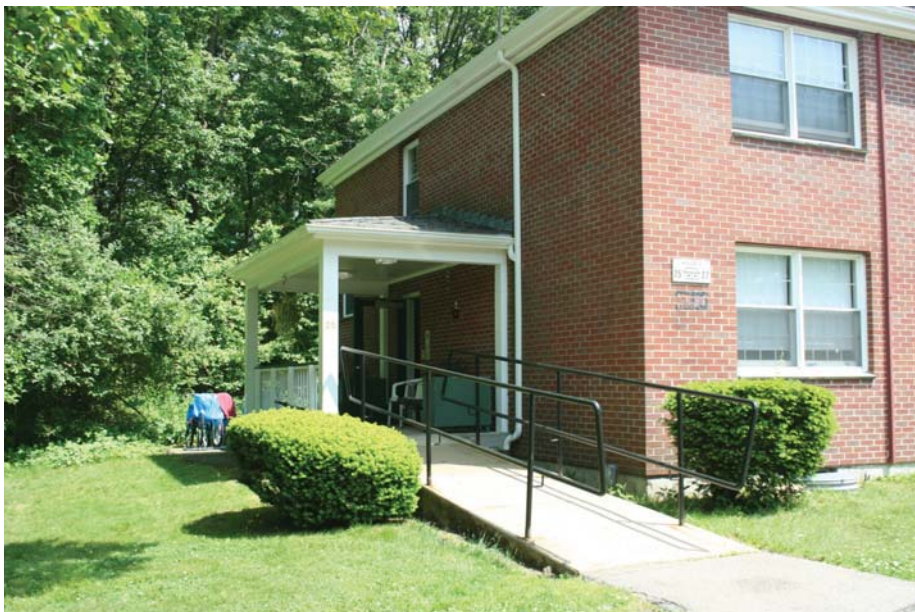
4. Entries on each end are similar- several steps up with a porch roof and railings. One entry at each building has a ramp up from grade that was not part of the original construction.
