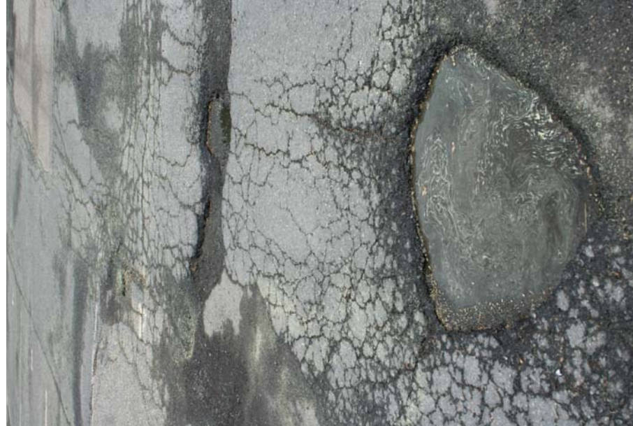
11. Paving is in relatively poor condition, especially in the parking areas. Walks are adequate but warrant ongoing maintenance.
