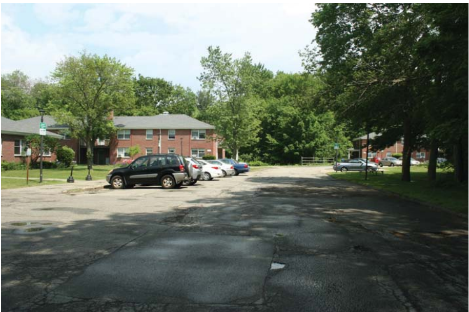
2. The spur road is a wide swath of asphalt in relatively poor condition. Parking spaces should be more clearly laid out so that the paving is used more effectively.
