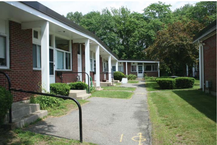
5. Overwhelmingly, apartments do not have accessible entries. Concrete stoops are several steps up from the walks in most locations. All of the 18 buildings have the same articulation and colors giving a sameness to every apartment, building and adjacent green space.
