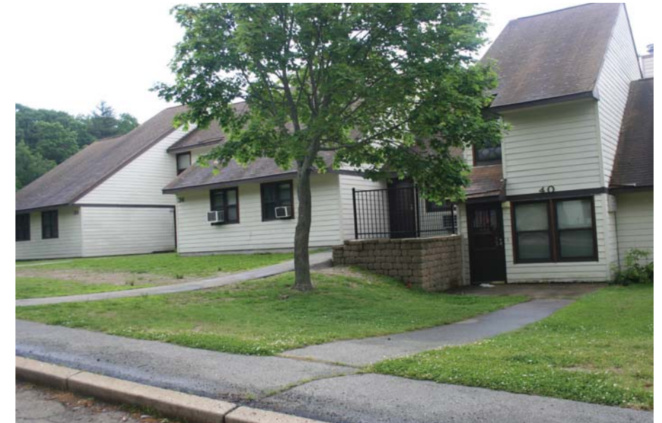
9. Most apartments are at grade with a roll in entrance. The sloping landscape is accommodated with occasional retaining walls where buildings step down along with the topography.
