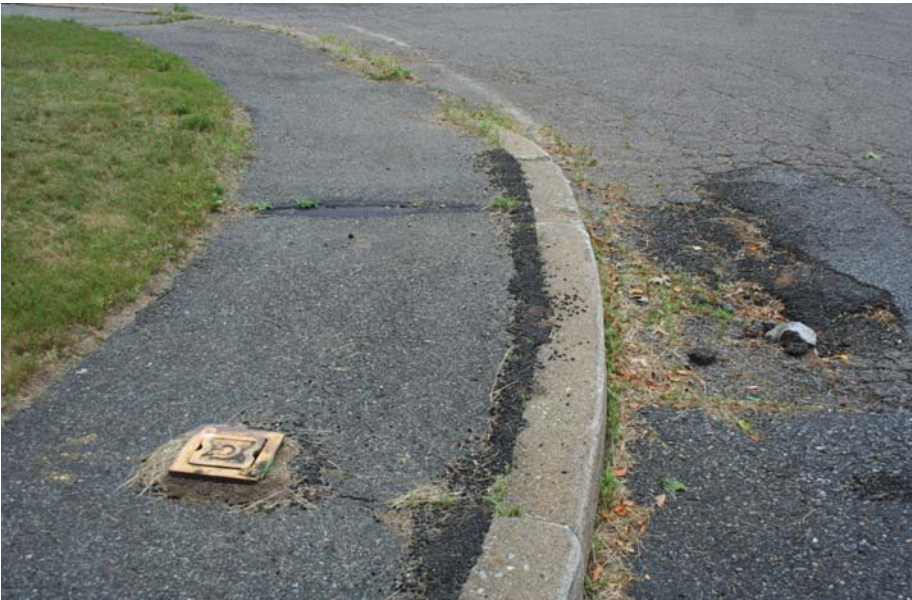
4. Curbs, sidewalks and streets are in relatively poor condition and do not adhere to all accessibility requirements. Most areas do have asphalt sidewalks adjacent to the street, acknowledging the importance of pedestrian safety for family housing.
