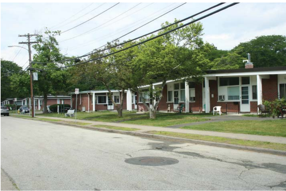
2. Half the buildings are oriented parallel to the street and half are oriented at 90 degrees, forming a kind of basket weave pattern in the overall layout. The brick buildings have overhanging roofs on both sides supporting by steel columns clad in white painted wood.
