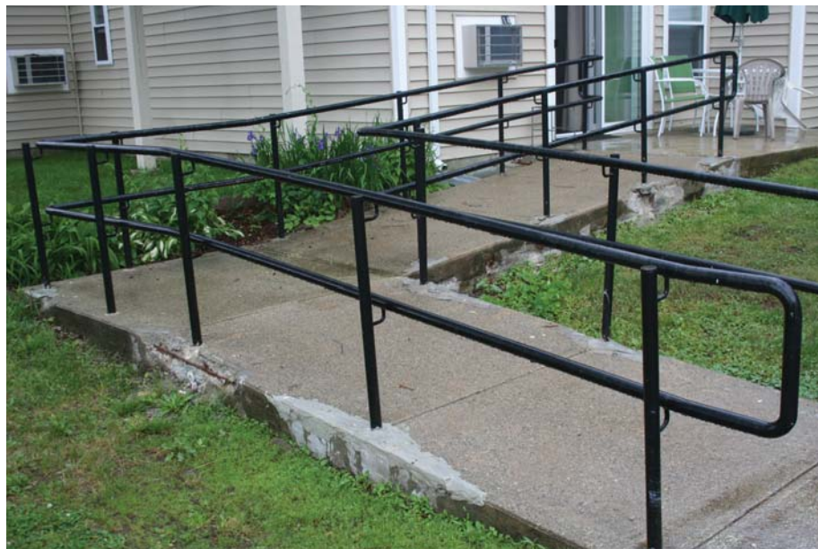
10. Ramps provide accessibility to some building entries and terraces. Many have been patched but are still in poor condition. Some could be eliminated with regrading of the site, making it more attractive and lowering maintenance costs.
