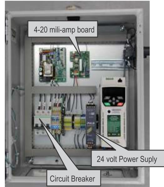
View of the variable rate controller, with Emerson variable frequency control
