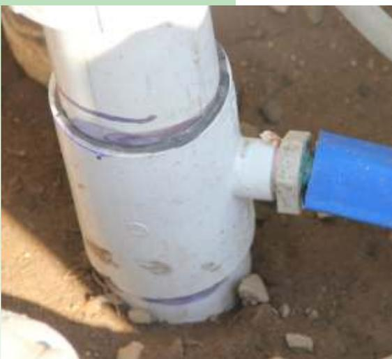
For new installations, a  $\frac{3}{4}$  inch threaded port is needed to insert the acid injection probe.
