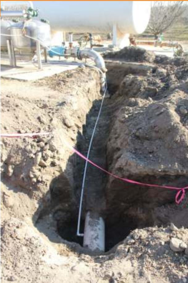
The grower or irrigation company will need to install a 1/2 inch PVC line, from at least one but preferably two elbows downstream of the point of injection of acid. Tap to be on the side.
