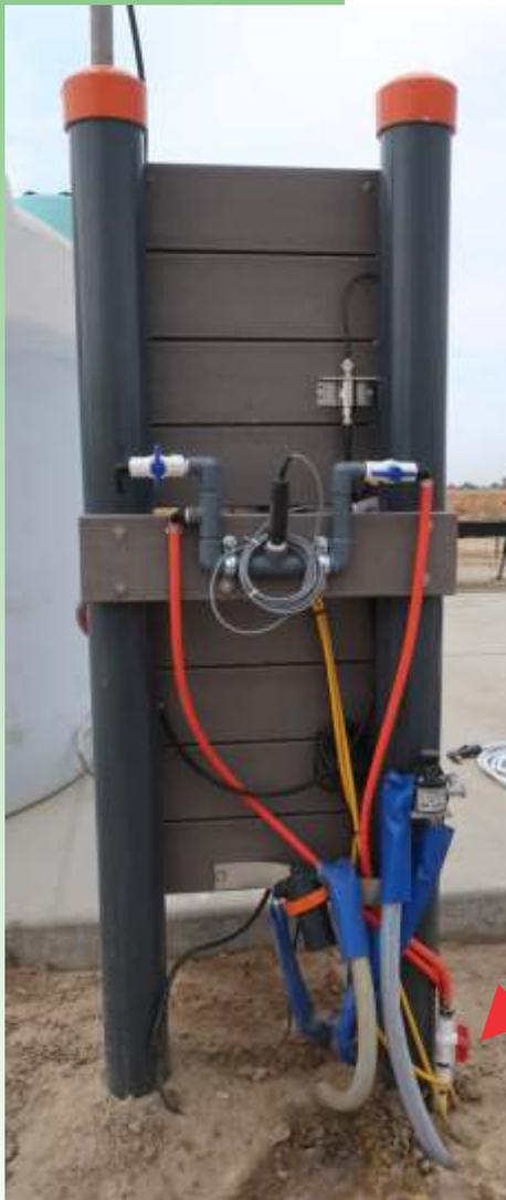
LED light on top of box is normally set to go on if pH goes up to 8, or down to 6. These set points can be programmed to different pH levels
