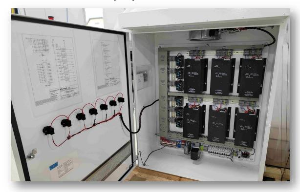
Induction Master Controller with Two Induction Power Modules, Lighting Old Style LEDline® with induction power connectors
