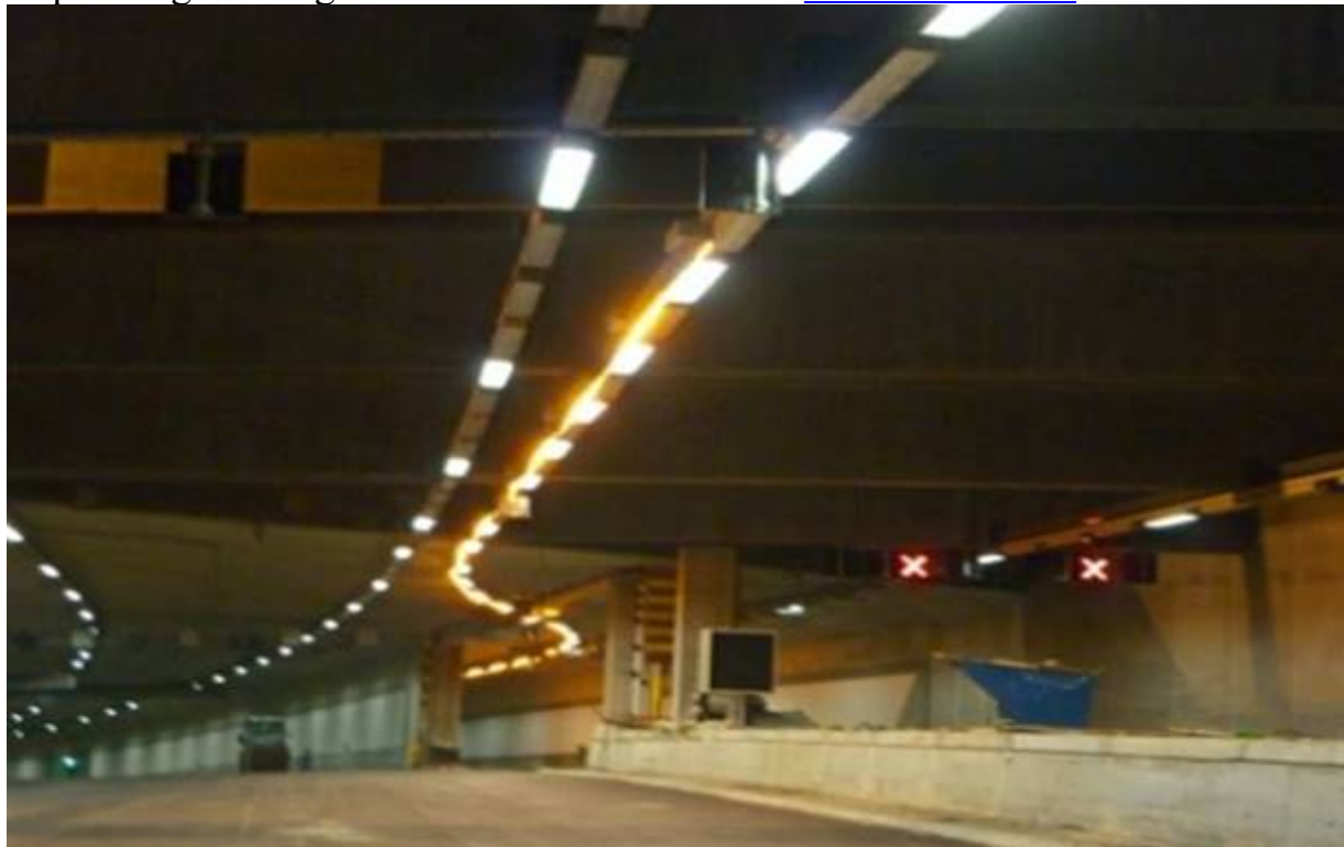
When a tunnel is blocked in the Bjørvika Tunnel Oslo, LEDline® is used as ceiling sequencing tunnel guidance for traffic. Video at www.ledline.net
