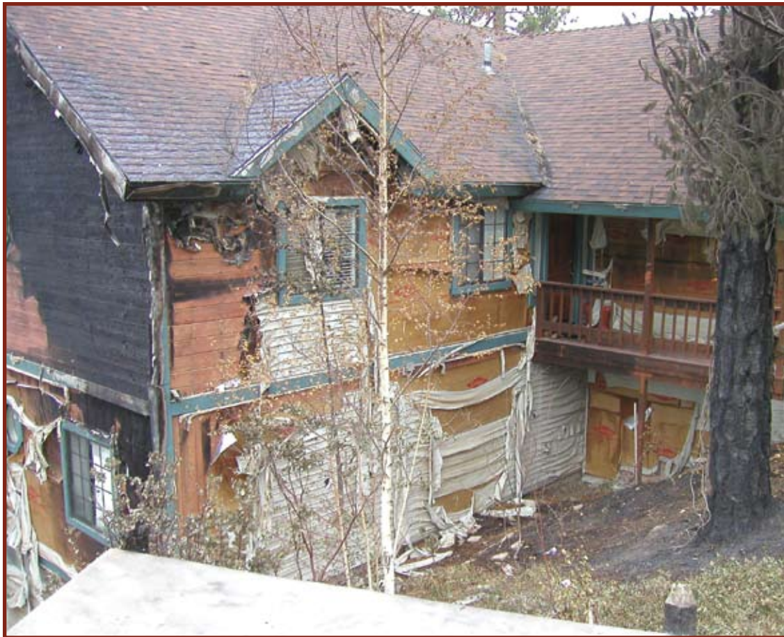
Figure 32. Home at 26150 Walnut Hills Dr. Thermal exposure from the destroyed home at 26142 contributed to the vinyl sloughing off. Surface fire burned the vinyl siding and under-layment on the northwest side (left) and worked its way up the wall burning the wood siding. Blackened asphalt shingles in the roof valley (center top) are from accumulated needles that burned.
