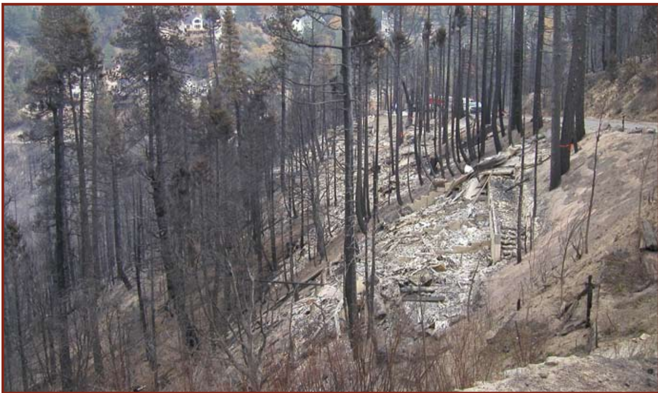
Figure 12. View to the east, principally of five destroyed homes on Trinity Dr. (971-949). The high degree of consumption of tree and shrub foliage downslope from these homes likely indicates high intensity flame exposure.
