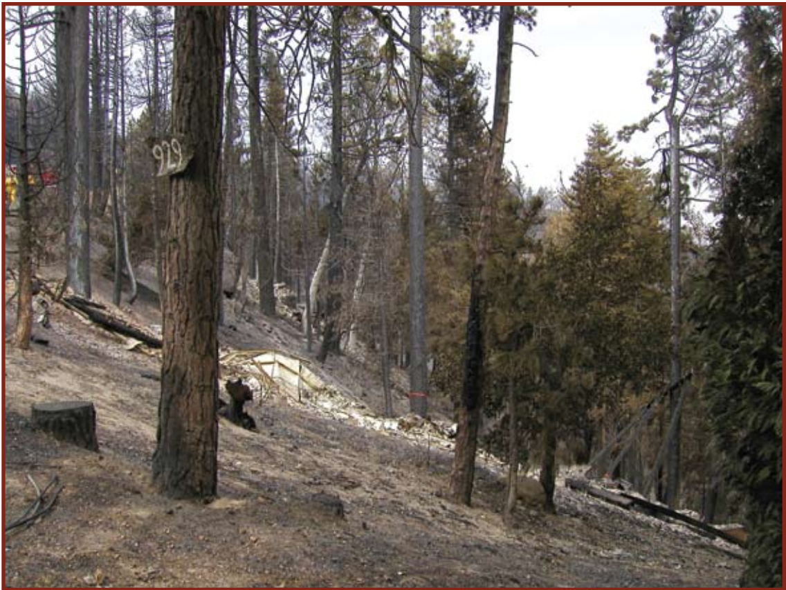
Figure 14. Destroyed home at 933 and 941 Trinity Dr. The low hanging, unconsumed canopy suggests that these homes were ignited from a surface fire and/or directly from firebrands.
