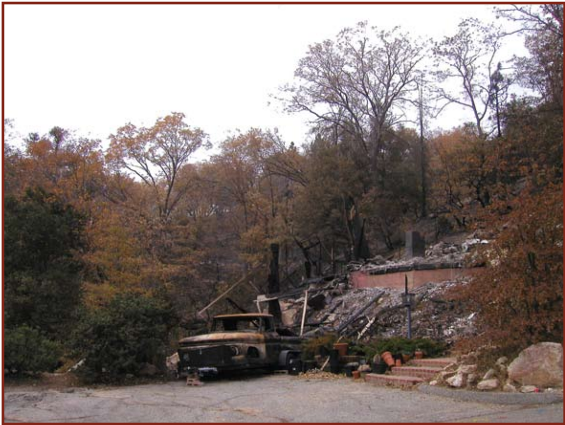
Figure 28. View of 710 Sonoma Dr. National Forest System lands are directly behind the destroyed home (west). The unconsumed vegetation surrounding the destroyed home indicates the likely cause was surface fire and/or firebrand(s). The neighboring house directly uphill survived (out of view to the right at 26516 Amador Ln.).
