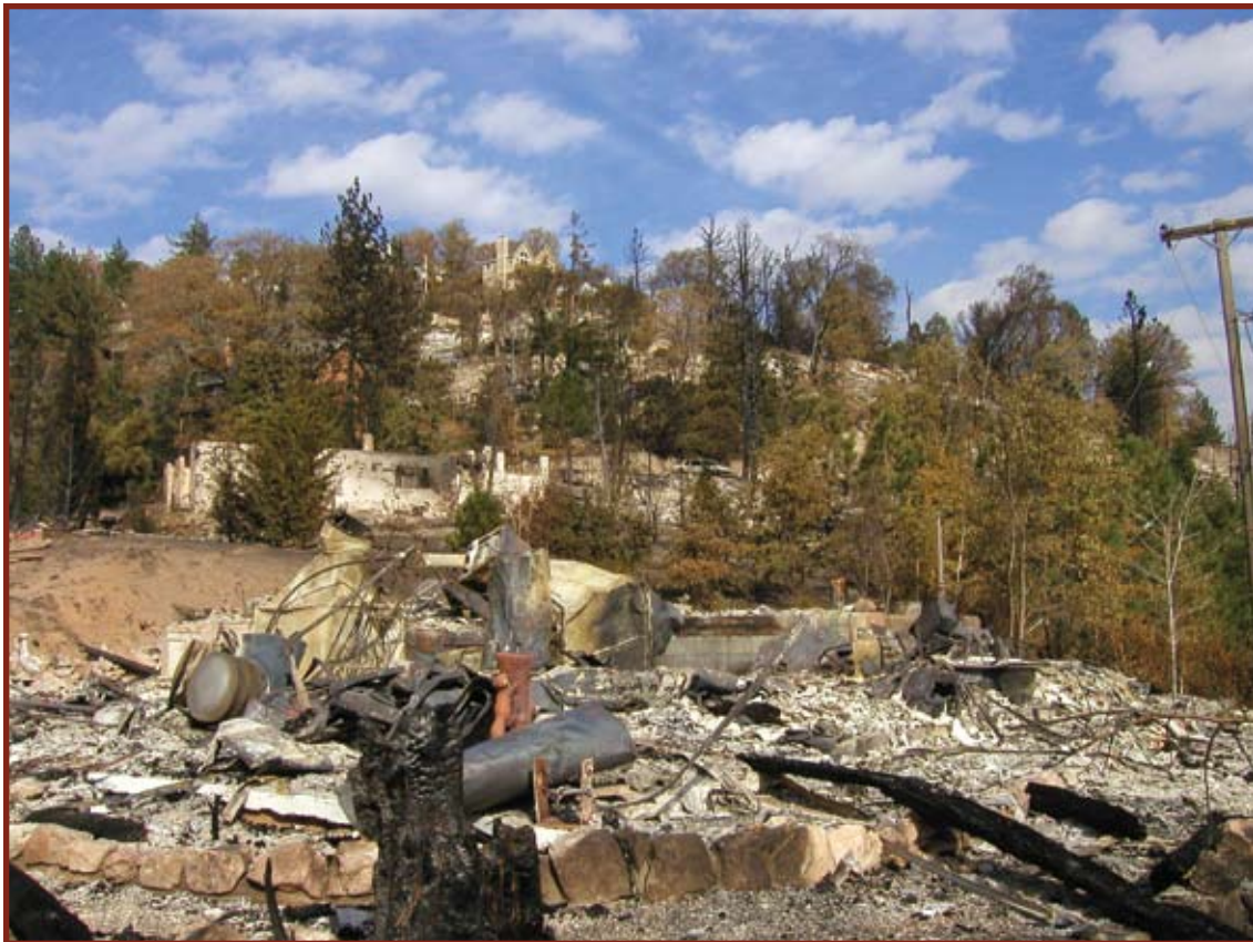
Figure 23. A view to the northwest upslope from 810 Marin Ln. through four levels of home destruction. The unconsumed vegetation between rows of destroyed homes indicates that a high intensity vegetation fire did not spread through the residential area.
