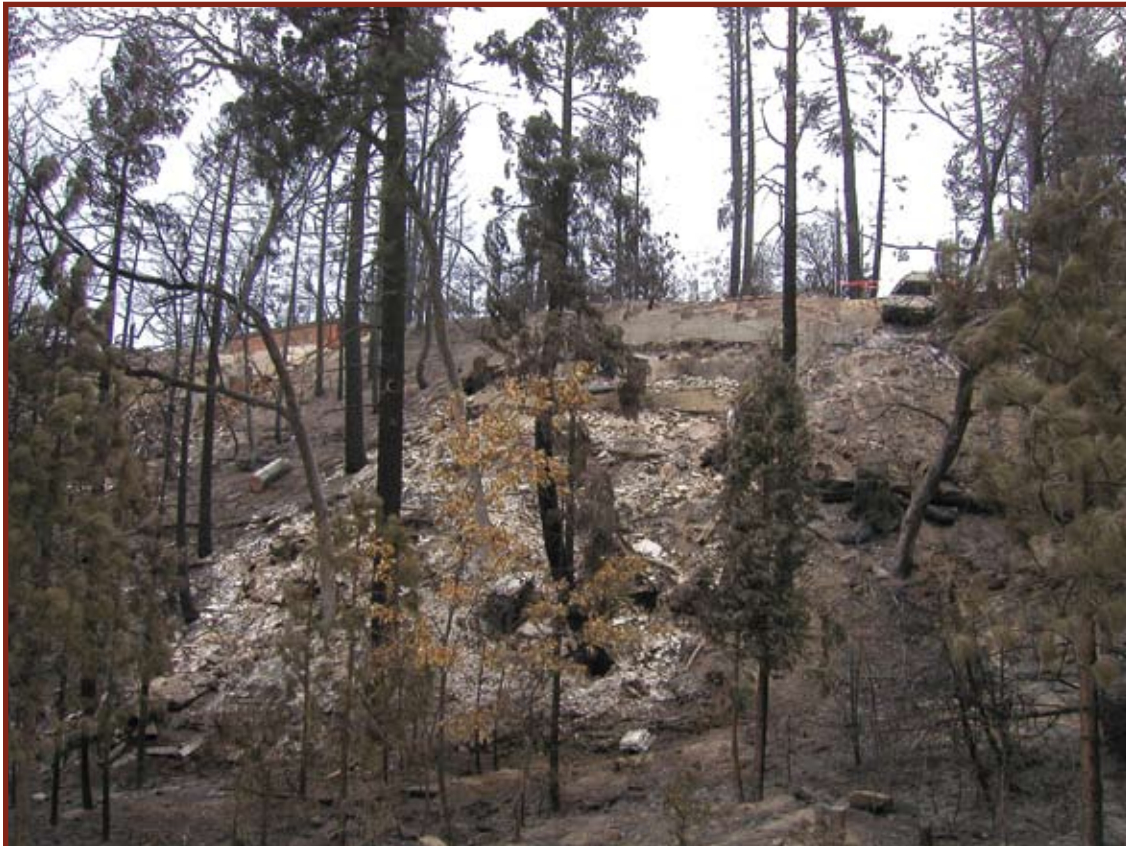
Figure 16. Photo of 26787 Merced Ln. from Trinity Dr. Note the steep slope (35-40°) with the remaining debris from the collapsed home spread down the hill.
